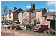
It demonstrates many of the features for which the Strutt farms are famous: the stone fire-proof construction of the ceilings and floors; the careful arrangement of feed storage for ease of delivery; and the use of natural ingredients allowing feed such as wet grains, cereals or hay to be tipped into pits or carted into stores that open into the first floor mixing room above the cow byres. The cow byres are well ventilated - another Strutt design feature.
