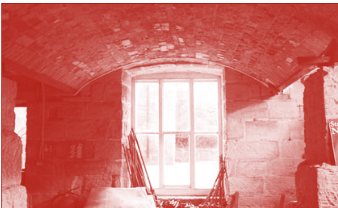
Picture of the brick arched ceiling
