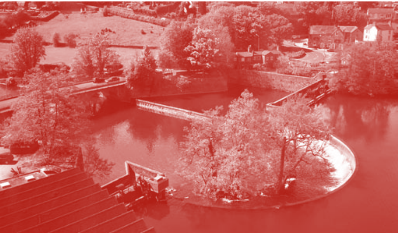
The Horseshoe Weir from the roof of East Mill
