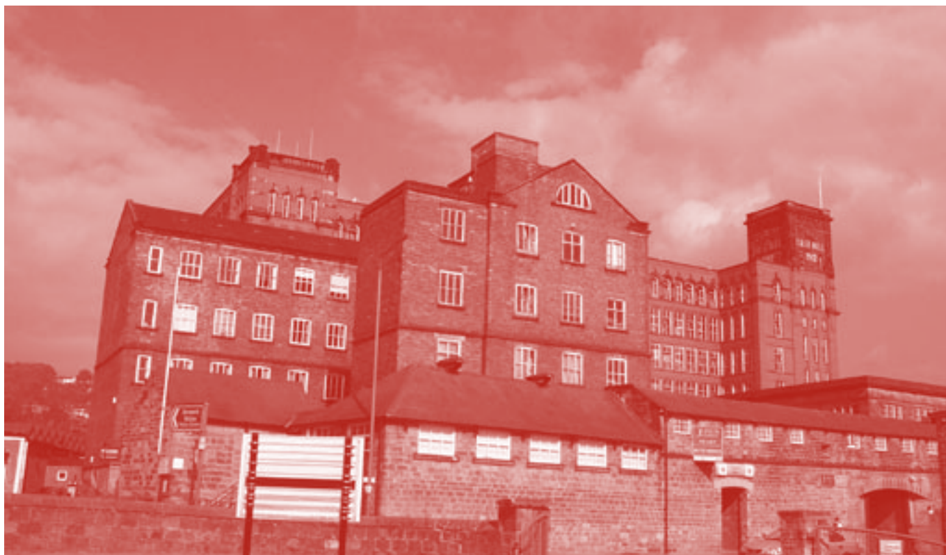
Strutt's North Mill with the East Mill behind
