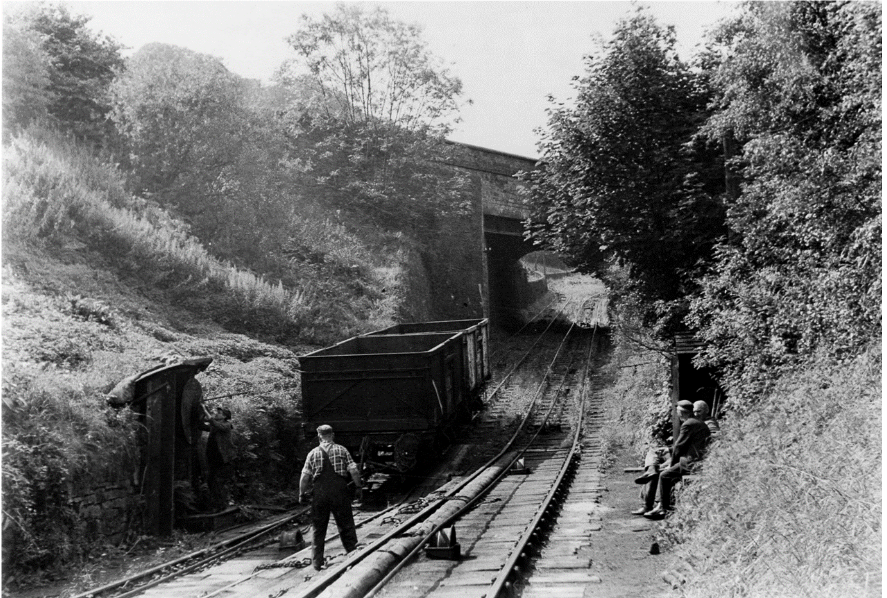
1966 – Indicator moved to the correct position as a wagon is about to ascend the incline
