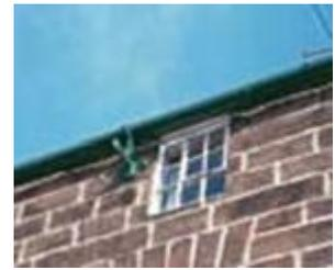
There are casements on the second floor. These are said to be Strutt designed and are nine-paned iron windows, four panes of which form each casement. It is clear that though they are of an early date they are not original. The first floor windows have voussoirs. Some modern alteration has taken place to the windows. On the rear elevation evidence survives of an original exit to the garden at half-landing level by means of a bridge.
