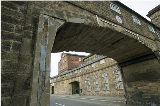
A sandstone bridge linking the two separate areas of the former Strutt Mills complex on either side of the Ashbourne Road. The archway also served a defensive role. Along its length are gun embrasures which protected the West Mill counting house.
