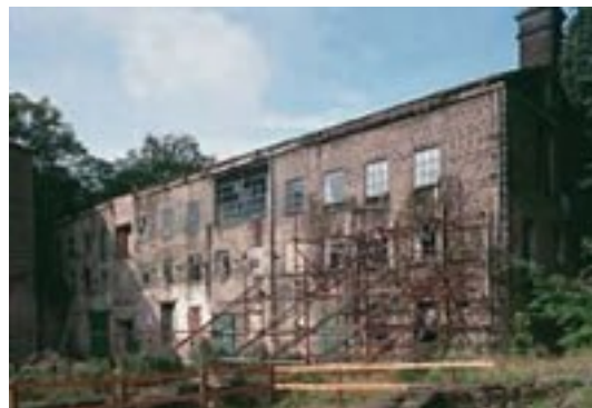
Cromford Mills awaiting repair
