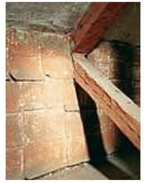
The attic floor is supported by a matrix of wooden beams, an arrangement quite different from any of the lower floors. The matrix is formed of transverse members every two bays (the tie-beams of the trusses) with four longitudinal members between and the beams are all clad in sheet metal. The irregularly spaced cast iron columns are secondary and thus this top floor was probably a clear space.
