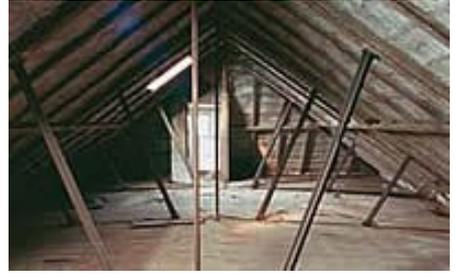
The West Mill is of particular interest. It is an L-shaped extension projecting from the middle five bays of Long Mill. Like Long Mill it is brick-built with a masonry ground floor but it is a storey lower and a passage leads from the fourth floor of Long Mill through a hip-slope to the roof space of West Mill.
