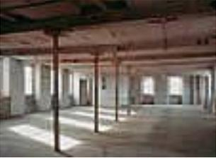
The floor below, in contrast, has a transverse beam each bay with a central rank of cruciform cast iron columns augmented by later round section cast iron columns. It is not clear that these columns are original, and taking into account the date of the reconstruction of the mill it is likely that they were added later. In July 1799 the Griffin Foundry in Chesterfield supplied 23 'iron pillars' but it is not clear which part of the mill these were for.
