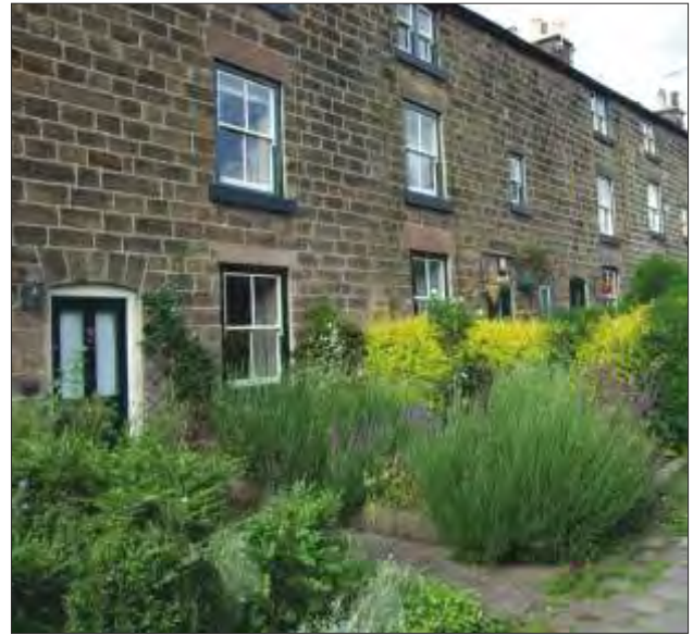
Fig. I.5 The northern terrace of Long Row, Belper, built by the Strutts between 1792 and 1797, provides an excellent example of the industrial housing constructed by the mill owners for their workforce. The houses in this row are of Derbyshire gritstone, with a continuous sloping eaves line, and have floor plans that interlock around the staircase (photograph: David Knight; © Trent & Peak Archaeology)
