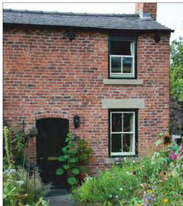
Fig. 4.43 Short Row, Belper: one of 47 red-brick terrace houses with slate roofs, built by the Strutts for mill workers around 1788. The development comprised four separate rows of mainly one-up, one-down cottages, all originally lacking piped water and other basic utilities (photograph: Mark Suggitt; © DVMP)
