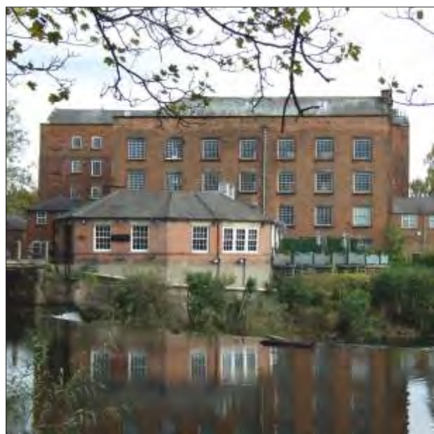
Fig. 4.28 Boar's Head Mill, Darley Abbey: west elevation of the West Mill, constructed from 1821, and in the foreground the mill's dining room, built probably in the 1820s or 1830s and since converted to a restaurant. 11 The Evans family's textile mill complex is now enjoying a new lease of life as the focus for a wide variety of small to medium industrial and other commercial enterprises and as a wedding venue (photograph: David Knight; © TPA)
