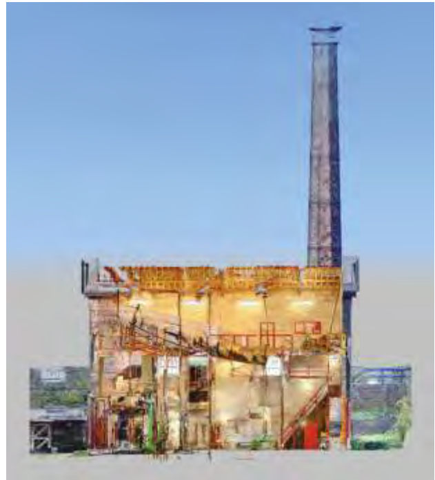
Fig. 2.1 Laser-scan rendering by the Heritage Lottery-funded Young Roots project 4 of Leawood Pumphouse on the Cromford Canal (source: Derbyshire County Council). Built in 1849, the pumphouse building accommodated a steam pumping engine that drew water from the Derwent to increase the supply of water to the Cromford Canal
