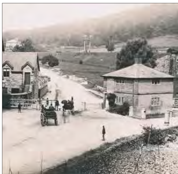
Fig.4.42 View northwards along the turnpike linking Belper with Matlock in a postcard of 1880, showing the Ambergate tollgate (right) at the junction between the turnpike and the road to Ripley (A610). The embankment of the railway from Derby to Matlock may be seen to the north of the tollgate (source: Adrian Farmer collection)
