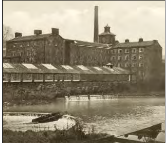
Fig. 2.2 View of the Milford mill complex, developed by Jedediah Strutt from the 1780s but demolished in the 1960s. The upstream weir was built between 1787 and 1792, while the weir in the foreground (with central fish ladder) was constructed before 1840. These and many other historic photographs of the Derwent Valley may be viewed on the Picture the Past website (RAP Co Ltd, c.1910; courtesy of Derbyshire Local Studies Libraries and www.picturethepast.org.uk ; DCHQ001437)
