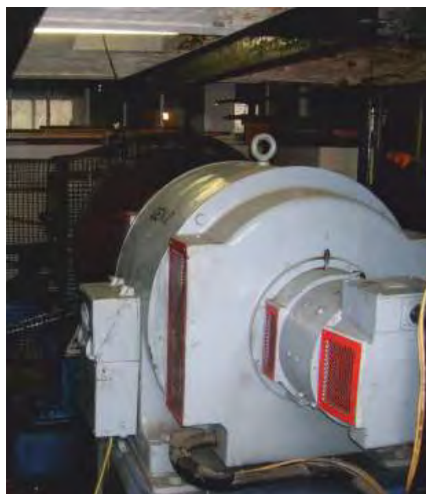
Fig.4.44 One of two hydropower turbines operating at Belper's East Mill, each with a capacity of 175kW. When in full flow, the power generated by both turbines is sufficient to provide 1,767,000 kWh per annum. Based upon current average rates of household energy use, this is enough to provide 535 houses with electrical power for a year (assuming 3,300kWh per annum for each house; photograph © Ian Jackson)
