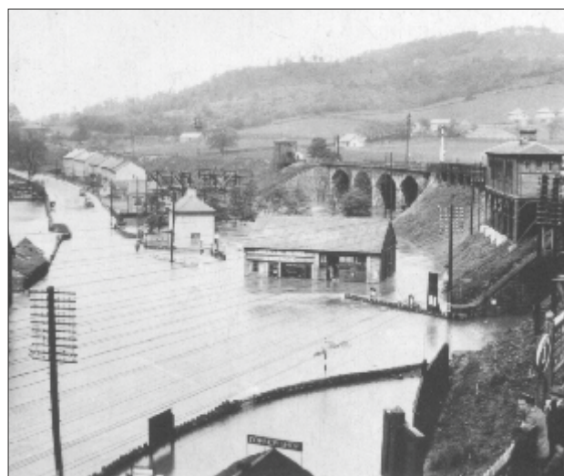
Fig. 4.54 The Great Flood of May 1932 caused significant damage to properties in Derby and elsewhere along the Valley. This photograph of the submerged junction between the A6 from Derby to Matlock and the A610 (right) is taken from broadly the same viewpoint as the 1880 photograph of the Ambergate tollgate (Fig. 4.42; photograph reproduced by courtesy of David Beevor)
