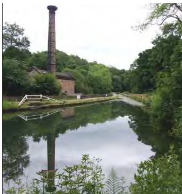
Fig.4.33 The Wigwell Aqueduct, visible in the distance, was built in the early 1790s by William Jessop with the assistance of Benjamin Outram and carried the Cromford Canal for almost 200m across the Derwent. The adjacent Leawood Pumphouse, constructed in 1849, housed a steam pumping engine to increase the supply of water from the river to the canal (photograph: David Knight; © TPA)
