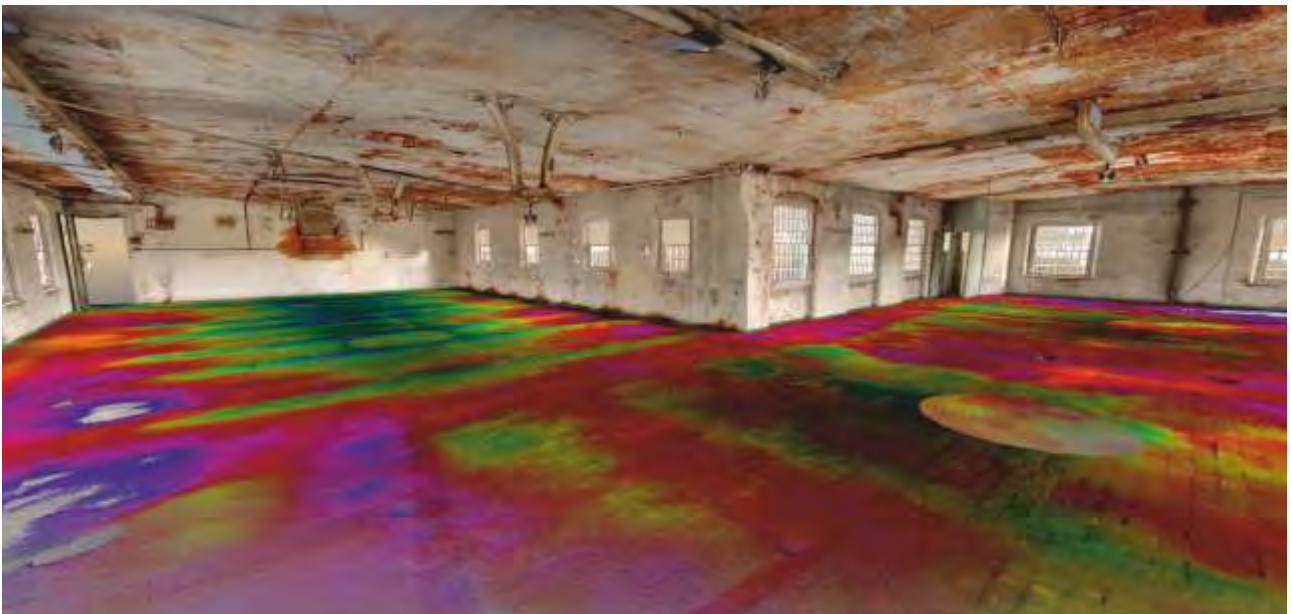
Fig.4.48 Boar's Head Mills: rendered laser-scanned point cloud of the third floor, coloured by elevation across a 7cm vertical range. The higher green and blue areas show where mill machinery once stood, while the lower red and magenta areas show eroded paths between machines (source: Derbyshire County Council)
