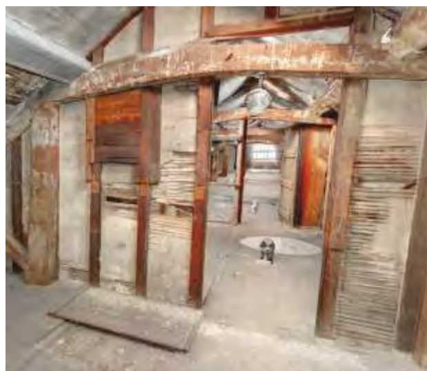
Fig. 4.40 Boar's Head Mills, Darley Abbey: the attic storey of the Long Mill, converted by the Evans family for use as a Sunday School in 1792, provides the earliest known example of its kind in the Derwent Valley. 9 This laser survey shows the condition of the building in 2014 (source: Derbyshire County Council)
