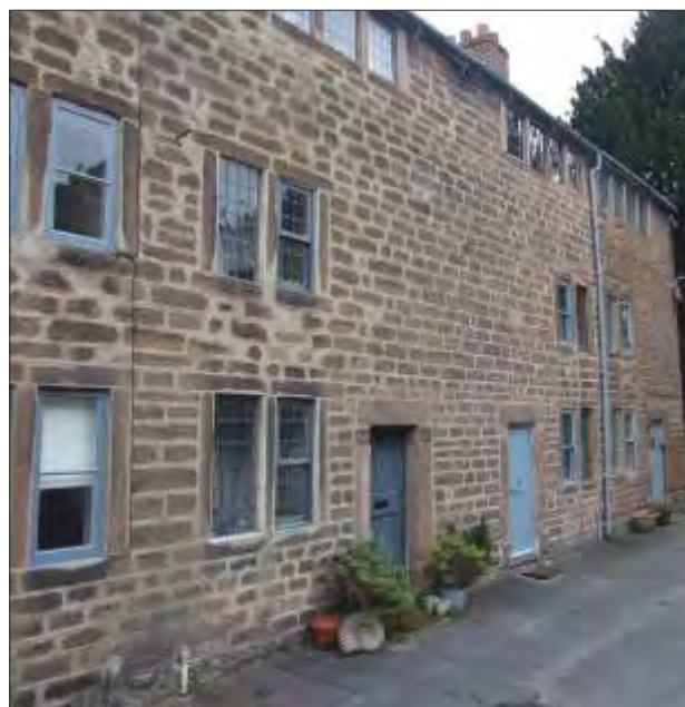
Fig.4.21 Three of the gritstone terrace houses on North Street, Cromford, which Arkwright built in 1776 for his mill workers and their families. Domestic accommodation was provided on the ground and first floors, while the top floor was employed as a workshop. The elongated third storey windows would have ensured sufficient light for home-based textile workers (photograph: David Knight; © Trent & Peak Archaeology)
