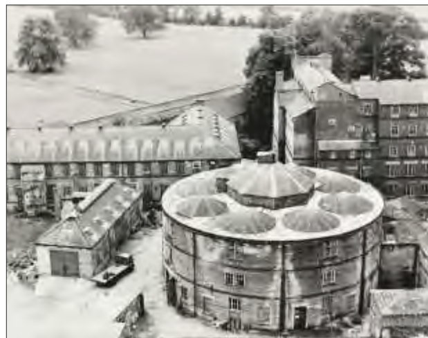
Fig. 4.35 William Strutt's unique Round Mill at Belper, photographed by A. N. Smith in 1959 shortly before its demolition in the 1960s. The panopticon Round Mill, built between 1803 and 1813, was designed according to the architectural principles developed by Jeremy Bentham. It was divided into eight segments, with an 'overlooker at the centre, like the spider at the heart of his web, [who] could see everything that happened in them' 9 (photograph © Derbyshire Record Office: Local Studies Library photographs)
