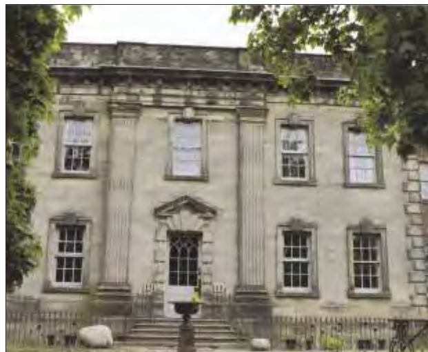
Fig.4.24 Front elevation of the younger Peter Nightingale's imposing house at Lea Hall, near Cromford, showing the classical frontage that he added in the mid-18th century to the original farmhouse. Recent documentary research 7 has demonstrated the pivotal role played by this wealthy landowner and lead merchant in the financing of Arkwright's cotton mills, workers' housing and associated infrastructure (photograph © Jane Middleton-Smith)
