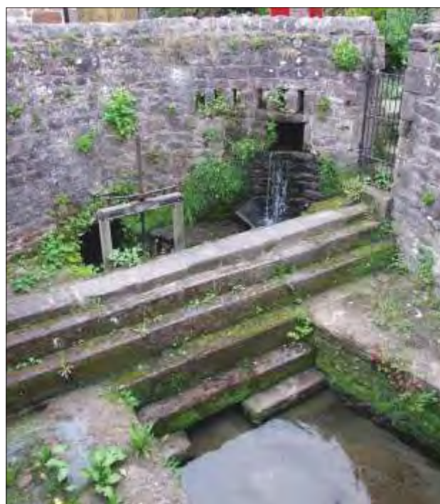
Fig.4.53 The 'Bear Pit', built by Arkwright in 1785 to allow access to the Cromford Sough. The sough was dammed and provided with a sluice that when closed enabled water to be diverted via an underground channel to enhance the mills' water supply (photograph: David Knight; © Trent & Peak Archaeology)
