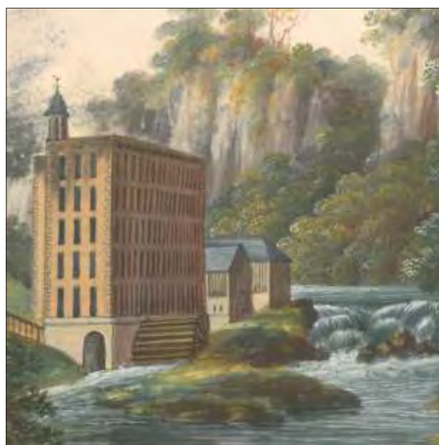
Fig. 4.22 Extract from George Robertson's watercolour of Masson Mill (c.1790) looking upstream along the limestone gorge between Cromford and Matlock. The building in the middle distance, adjacent to the weir across the fast-flowing Derwent, is thought to be Masson Paper Mill. The latter was built in 1770, some 13 years before Masson Mill, and was influential in the siting of the later cotton-spinning mill (© Derby Museums Trust)
