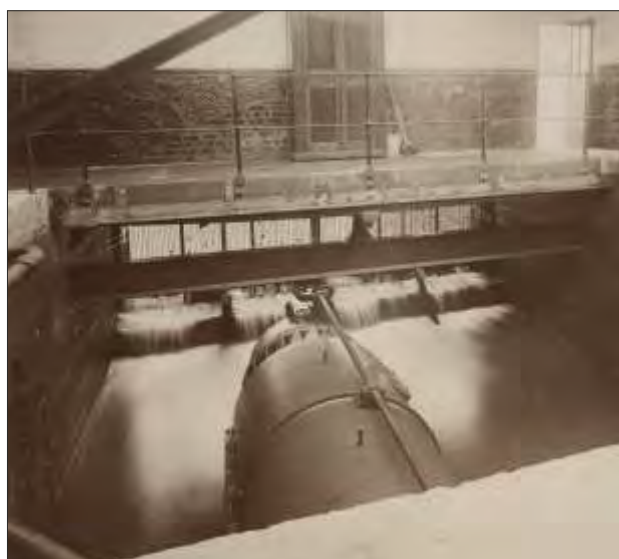
Fig. 4.59 View of water turbine in the demolished Milford Mill, photographed c.1907 (© Derbyshire Record Office: D3638-59). The turbine pit and supporting beam shown here may still be seen in the garden of the Mill House public house
