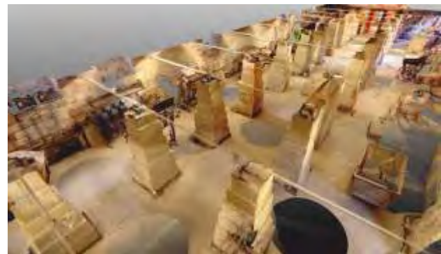
Fig. 4.26 Laser survey of the fire-proofed basement of North Mill, showing the rows of stone piers that carried cast iron columns supporting the floors above (source: Derbyshire County Council)
