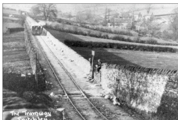
Fig. 4.41 Field survey and documentary research by members of the Butterley Gangroad Project 9 has shed important light upon the development of this early railway, built in the 1790s as a feeder line between limestone quarries at Crich and the Cromford Canal and closed in 1933. This 1930s postcard shows the mid-19th century Fritchley embankment (reproduced by courtesy of Derbyshire Archaeological Society)
