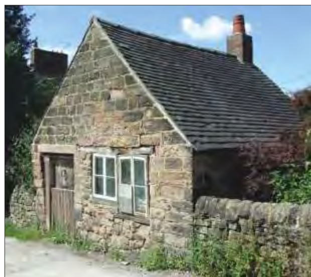
Fig.4.36. 8 Joseph Street, Belper: a rare survival of the nailshops that would once have been familiar features of the townscape. This building dates from the early 19th century, and was constructed of coursed gritstone with tile roof, brick chimney and cast iron windows (photograph: David Knight; © Trent & Peak Archaeology)
