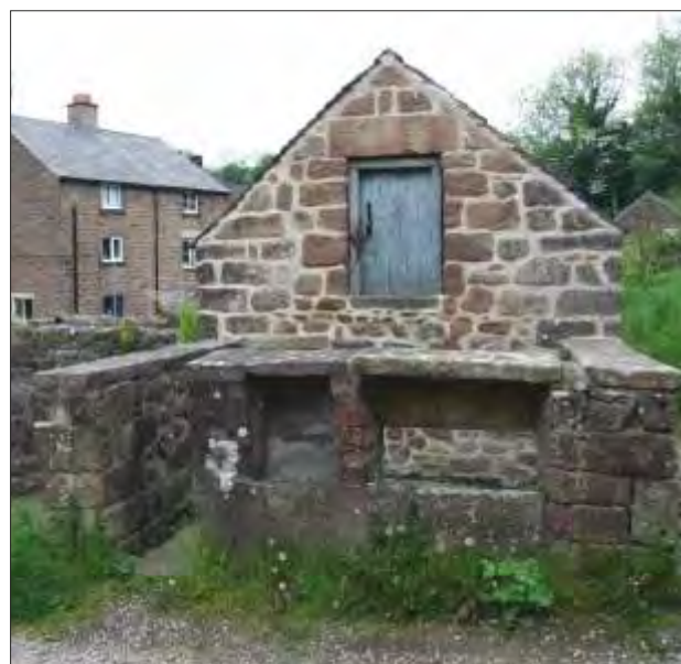
Fig.4.46 Swift's Hollow, Cromford: late 18th or early 19th century pigcote, incorporating a shelter and an open area for exercise with feeding troughs (photograph: David Knight; © TPA)
