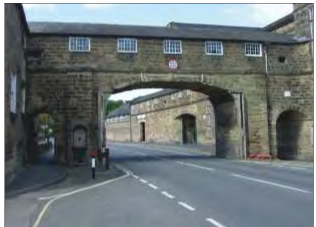
Fig.4.34 The Strutt family's concerns about social unrest, and in particular the security of their West Mill counting house, are demonstrated by the addition of gun embrasures either side of this arched footbridge, built c.1795 to link Belper's West Mill (left) with other factory buildings. Another embrasure was positioned above the arch on the other side of the footbridge (photograph: Adrian Farmer; © Derwent Valley Mills Partnership)
