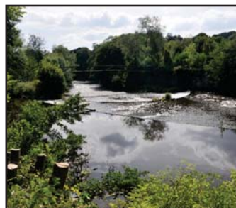
RESTORED: View of Milford Weir from Makeney Road after tree work was carried out.
