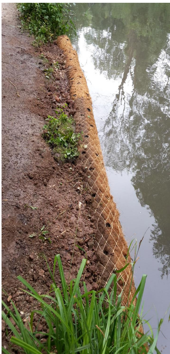
Coir Rolls after installation
