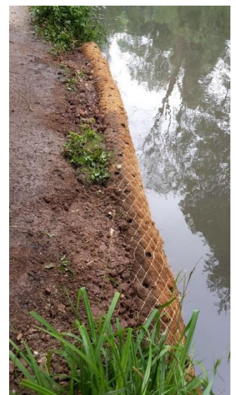
Coir rolls installed into canal banks
