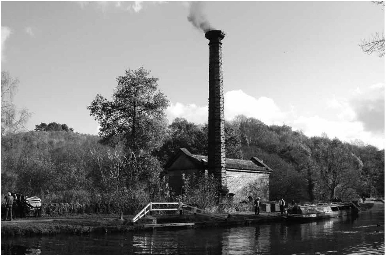
Leewood Pumphouse on the Cromford Canal
