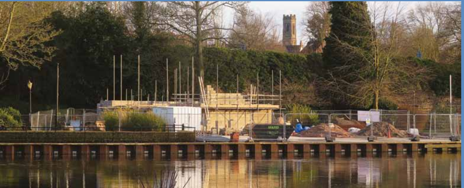
Building of the new tearooms, Belper River Gardens
