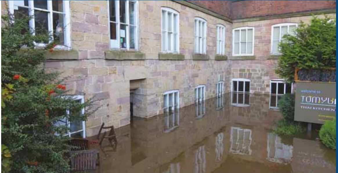
Flooding at the Belper Mill Complex, 2019
