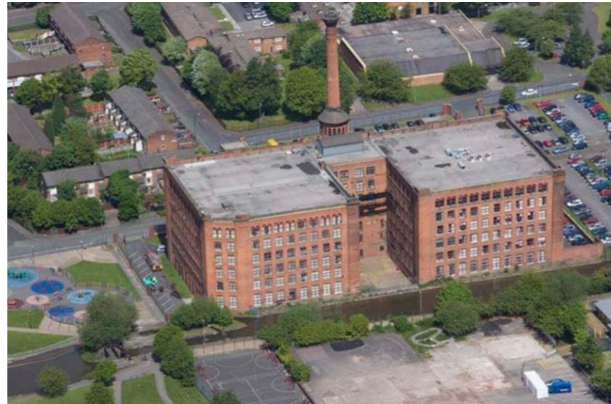
VICTORIA MILL, MANCHESTER
