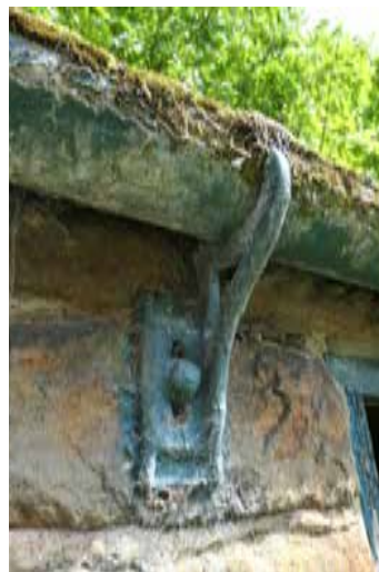
Fig. 62: An adjustable cast iron gutter bracket.
