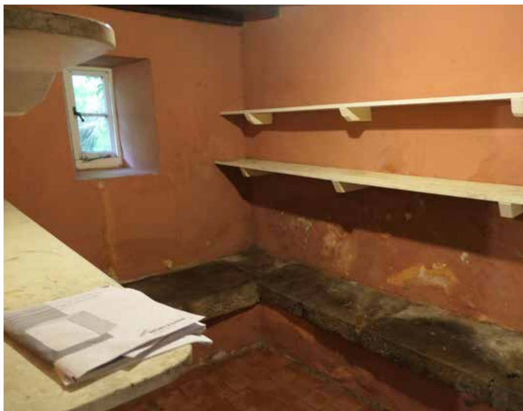
Fig. 22: The bullnose profile masonry opening and simple rounded kneelers below the opening are typical of those found in other farmhouses of the Strutt estate.
