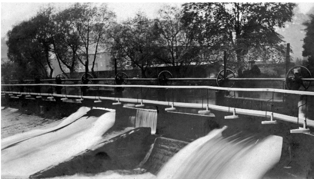
12. Darley Abbey Sluices and weir
