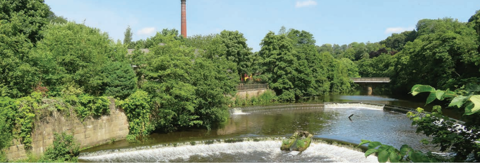
The weirs, bridge and mill chimney at Milford.
