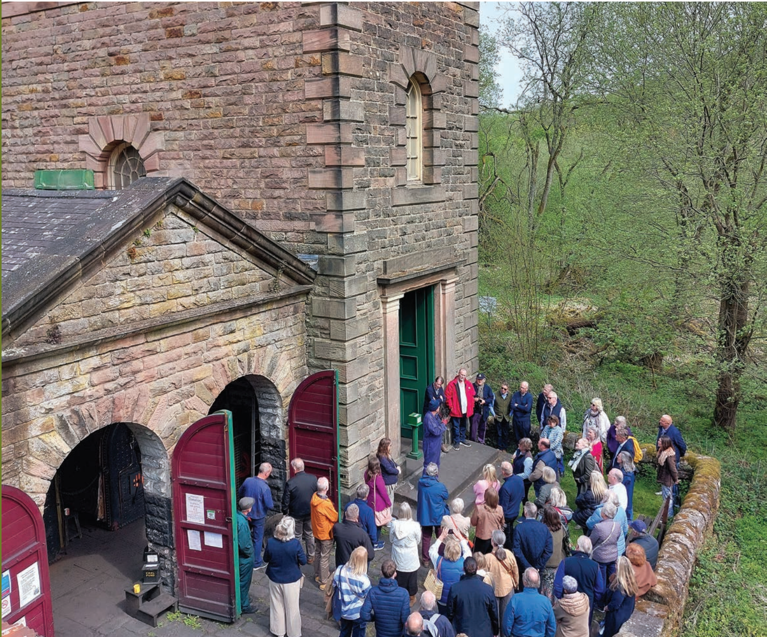
A group visiting Leawood Pumphouse on the Cromford Canal
