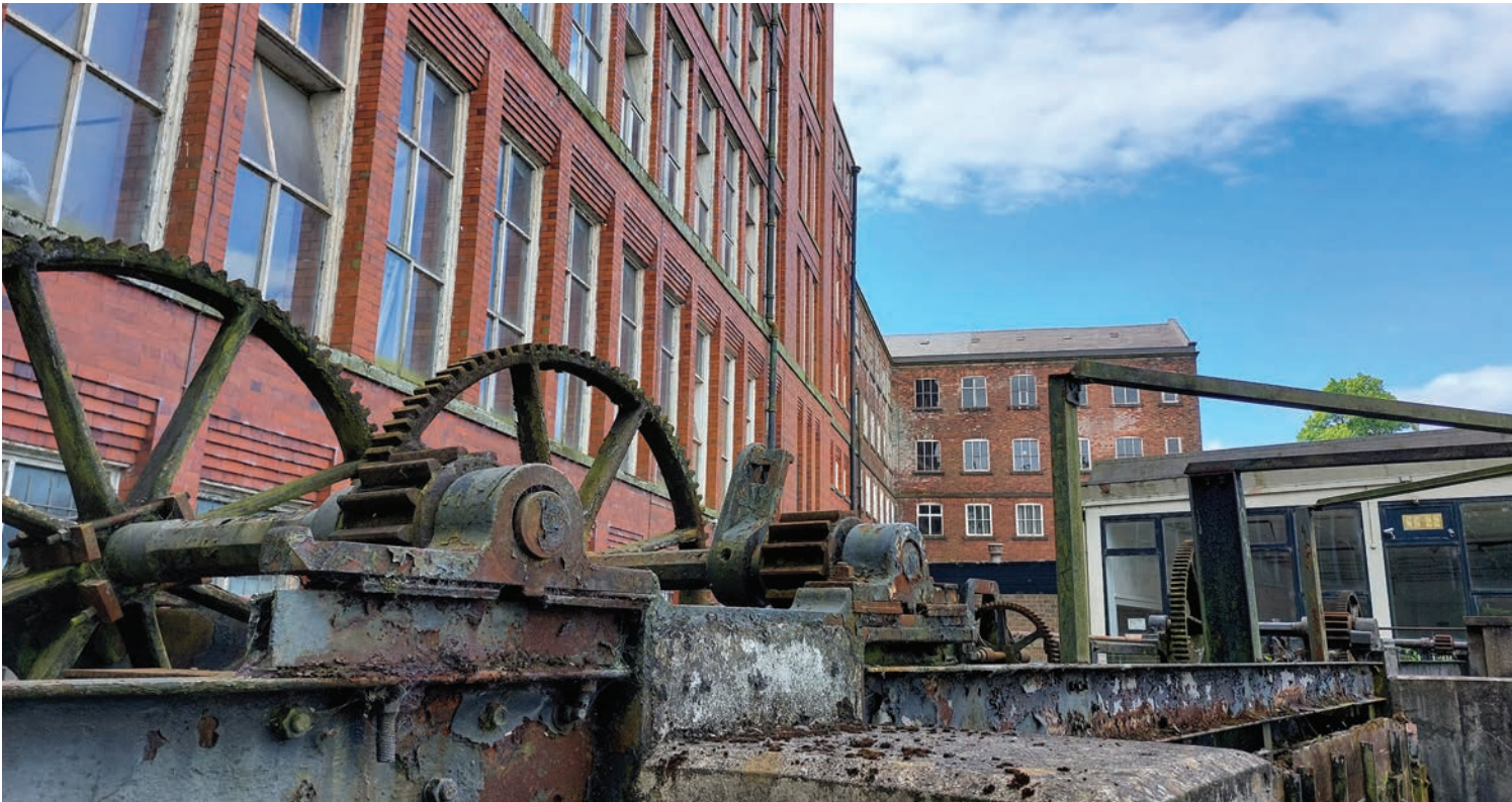
Belper’s East and North Mills
