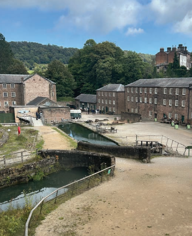
Cromford Mill Yard, looking towards the remains of the Second Mill
