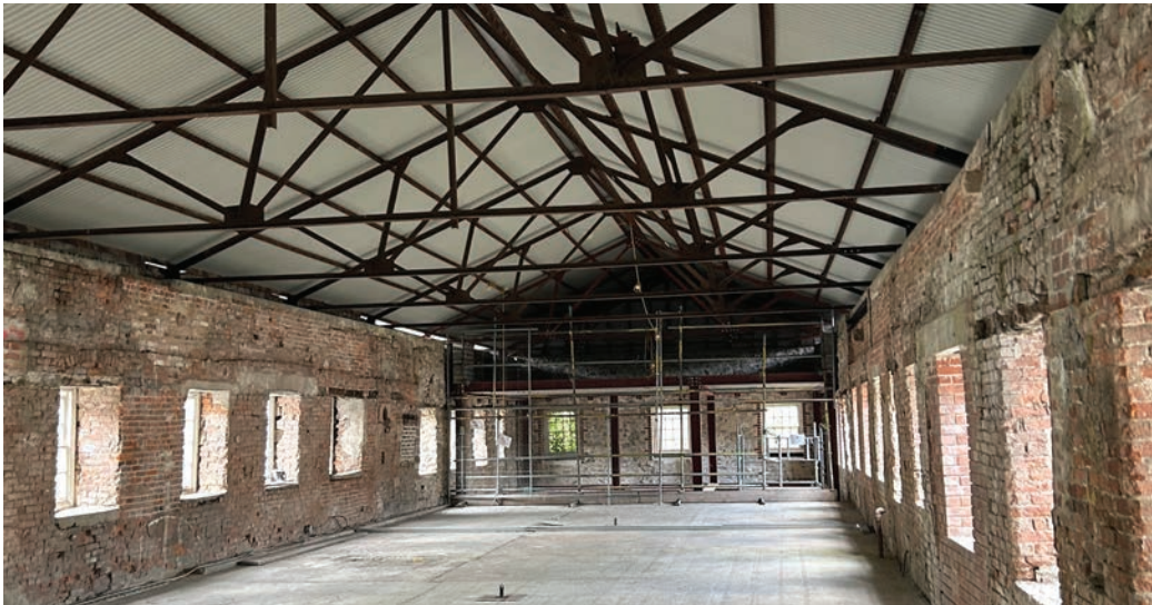
Arkwright’s first mill at Cromford - newly re-roofed in 2025
