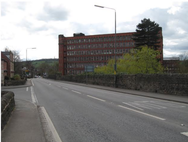
Belper's East Mill from the A6 looking south.
