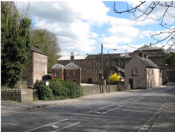
Cromford Mill from Mill Road.
